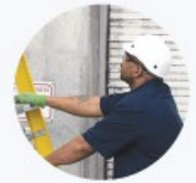
Face the ladder while climbing it
