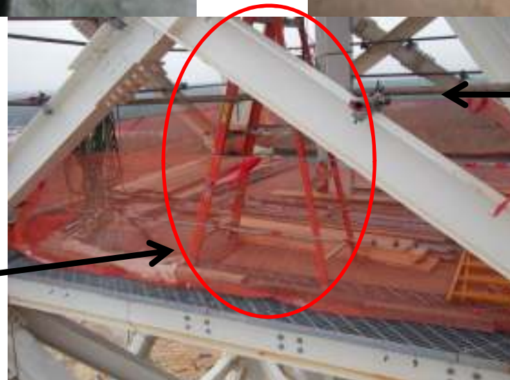
Additional guard rails installed to prevent falls off the Test Stand
