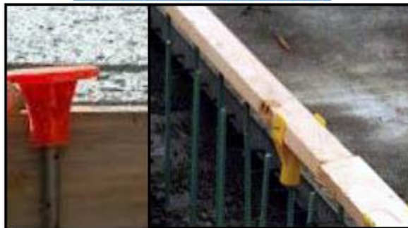
Steel Rebar Guard or Covering
