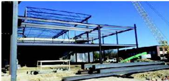
Figure 1. Integrated Engineering Services Building Second Floor Decking
