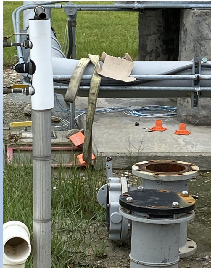
Synthetic sling left in the weather.
