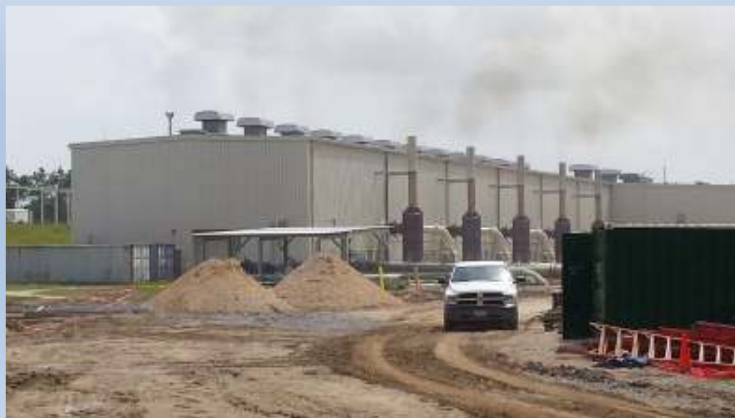
Building 4400 supplying HPIW, July 2, 2015
