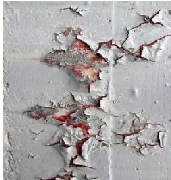
Flaking/Peeling Paint
