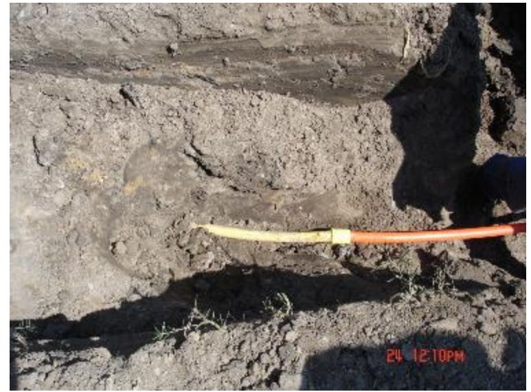
View of Repaired Section of Plastic Low Pressure Gas Line
