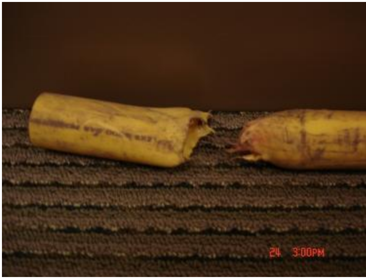
View of Damaged Section of Plastic Low Pressure Gas Line
