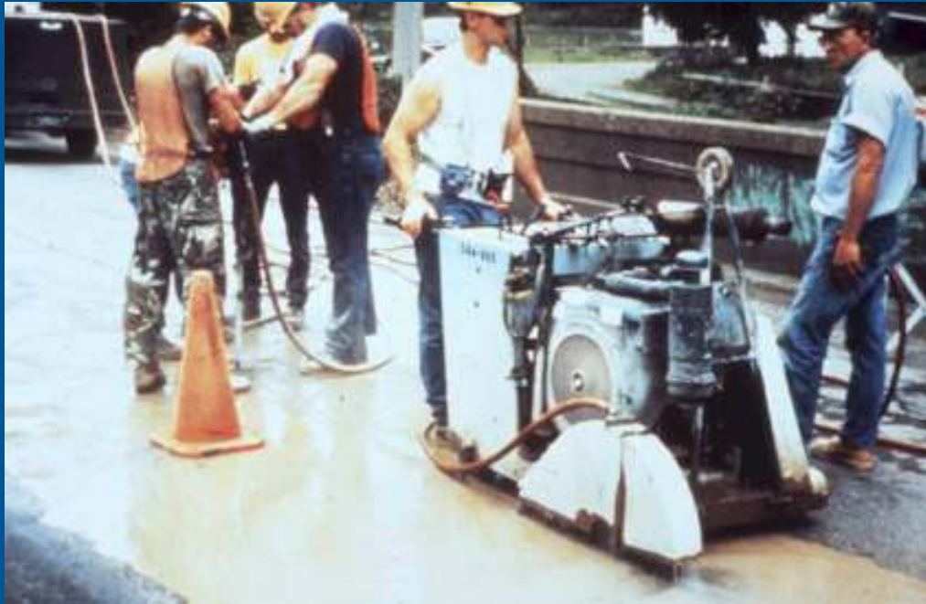
Using water to cut concrete and bricks
